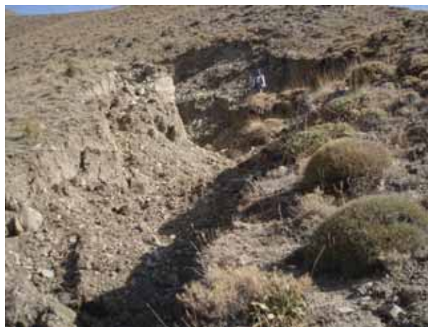
Figure 14 Bajebaj-Choupanlar road rock slide scarp
