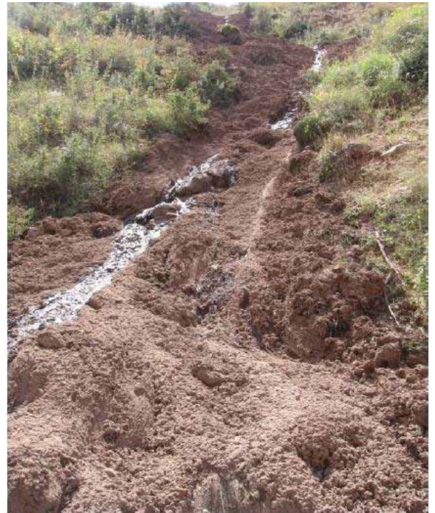
Figure 12 Soil flow near Bajebaj-Choupanlar road (zare et al. 2012)
