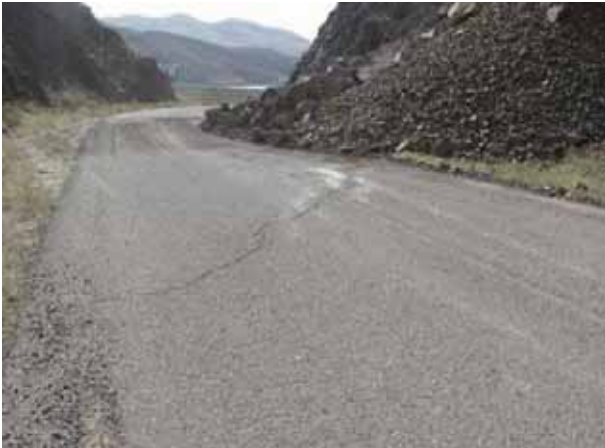
Figure 5 Rock slide in the Sattar khan Dam access road (zare et al. 2012)
