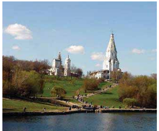
Figure 7. Museum - reserve "Kolomenskoye". Common view . Landslide slope.
