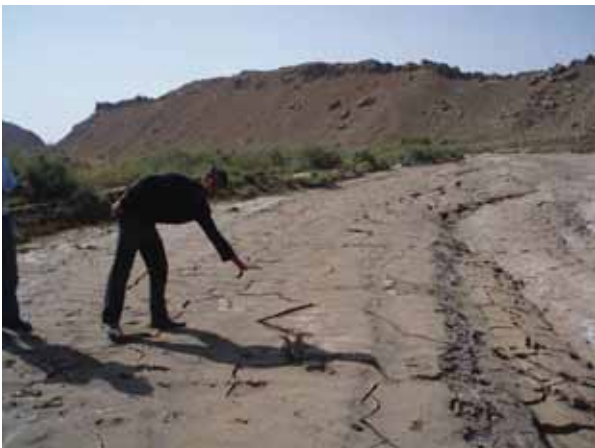
Figure 11 Lateral spreading in Nosham plain near Gamand Village with 0.5 meter settlement of the river bank
