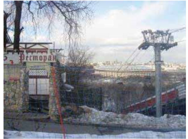
Figure 6. Place of landslide activation near ski jump.
