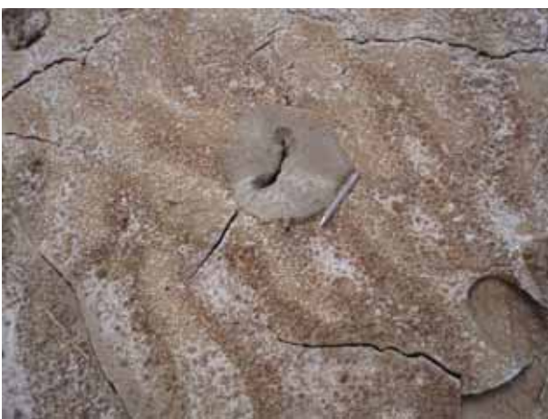
Figure 16 Liquefaction in the vicinity of Marjanlar village
