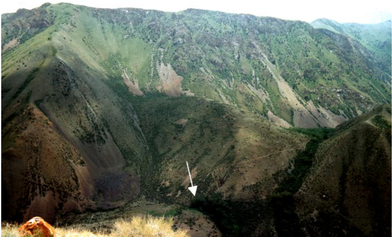
Figure 73. Kaskasu rockslide dam
