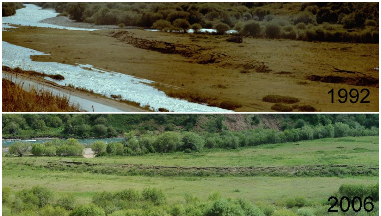
Figure 16. Surface rupture (reverse fault) of the M 7.3 Suusamyр earthquake Above, photo made in August 25, 1992, few days after the earthquake. Below – left part of the same scarp in 2006, 14 years later
