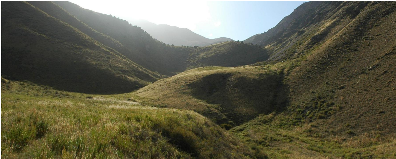
Figure 127. Northern Karakungey rock avalanche Compact blockage with convex slopes at the background and rock avalanche termination at the foreground. Note that rock avalanche body fills the valley only partially
