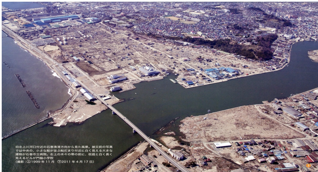
Figure 4. Ishinomaki city is one of the most severe damaged area. Several thousand houses outflow by huge tsunami and the litter accumulate at the foot slope of upland.
