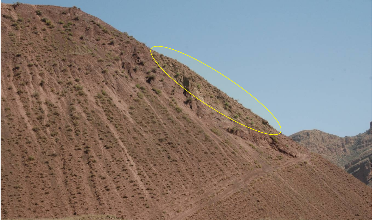
Figure 57. Patch of rockslide debris on the left outlet of the headscarp
