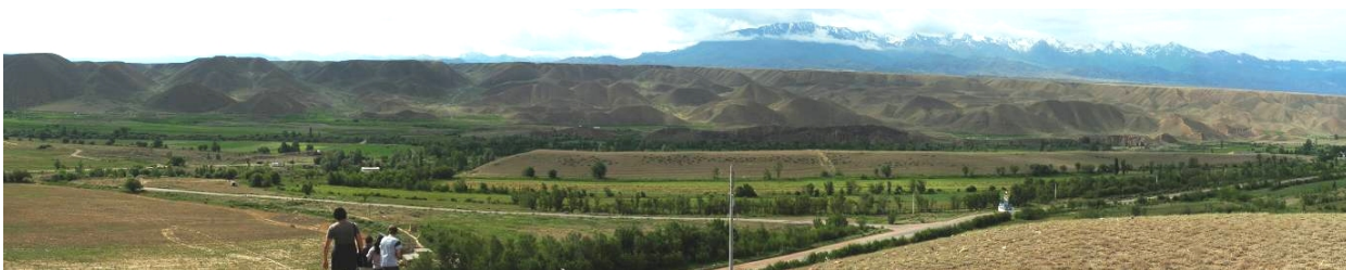
Figure 195. Panoramic view of the Chaek landslide
