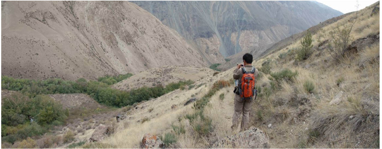
Figure 64. View on the lower widened part of the Kashkasu rockslide dam from the path crossing its upper part (see Figure 63)
