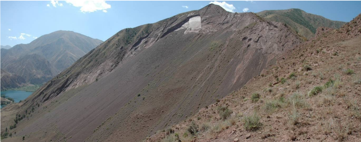
Figure 55. Right side of the headscarp coinciding with bedding where subsequent failures have occurred
