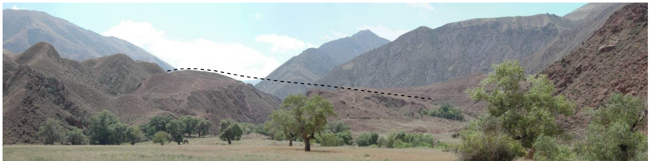
Figure 59. View on the Ak-Kiol rockslide dam from the downstream Dashed black line shows the assumed initial dam's crest profile, before deposition of the proximal part of debris
