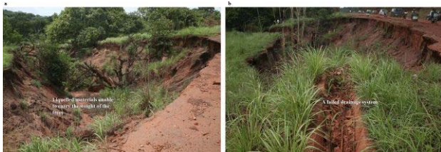
Figure 12 Effect of a blocked drainage on mass failure
