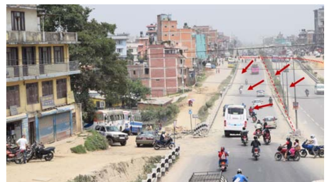
Figure 2 Road settled due to the landslide.
