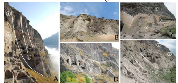
Fig. 3 Slope failure type and processes affecting the rocky cliff of Vardzia. (A) Large roto-translational rock slide involving both layers 1, 2 and 3. (B) Rock fall scarp in the upper part of layer 1. (C) Wedge failure at the contact between layer 1 (on top) and layer 2. (D) High and low angle potential planar rock slide. (E) High and low angle potential planar rock slide.
