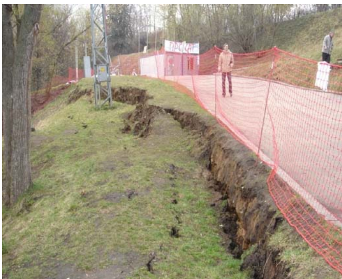
Figure 2. Landslide formed in Quaternary deposits in 2006.
