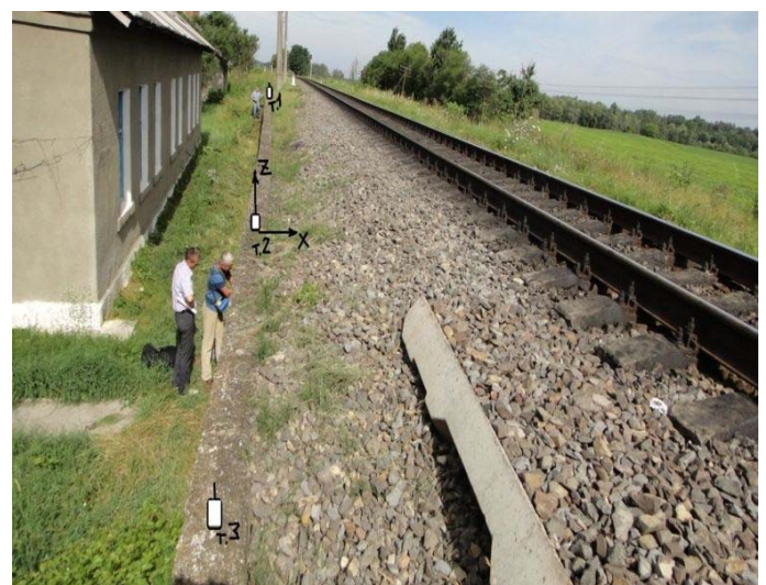
Figure 1 Location of vibration pickups during the inspection of the retaining wall.
