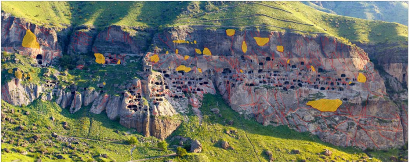
Figure 4. Unstable blocks and joints and open cracks in the Vardzia cliff
