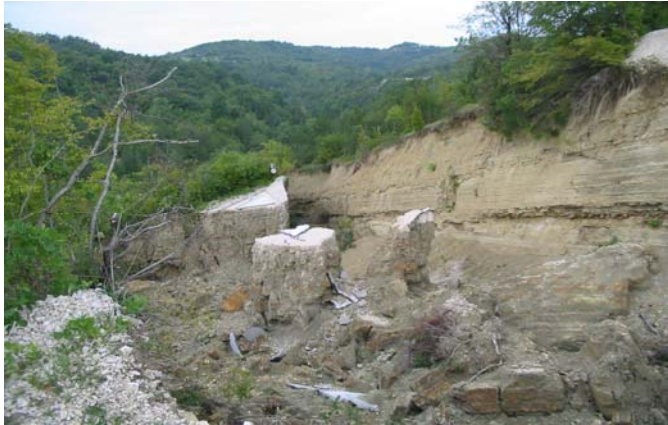
Figure 5 Atypical block slide developed in flysch-like rocks in Istria which belongs to “Gray Istria”. The trigger was heavy rainfall in 2004 (Arbanas et al. 2010)
