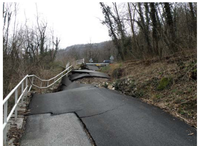
Figure 4 Valići Landslide developed in flysch-like rock in the Rječina River Valley. The cause was heavy precipitation in February 2014 (Mihalić Arbanas et al. 2017)
