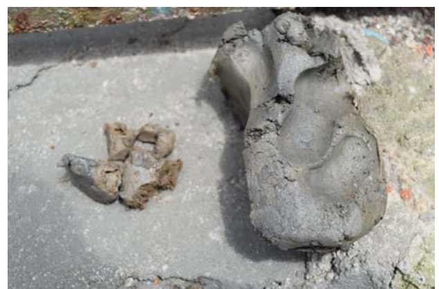
Figure 6 Soft clay observed at the site.
