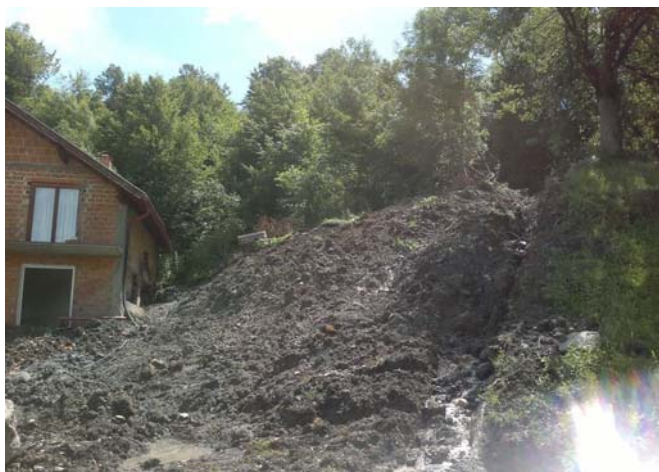
Figure 7 Landslide Lukavica-Prnjavor, Gračanica Municipality, BIH (photo by A. Džindo, 2014)
