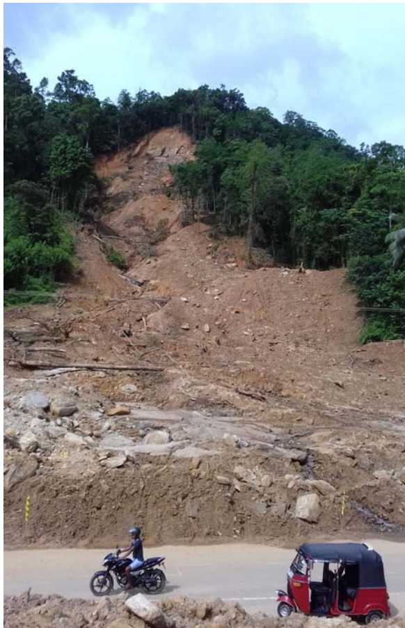
Fig 2: May 2017 Athwelthota landslide in Kalutara District Sri Lanka, which killed 09 people. Landslide was initiated from residual soil origin.
