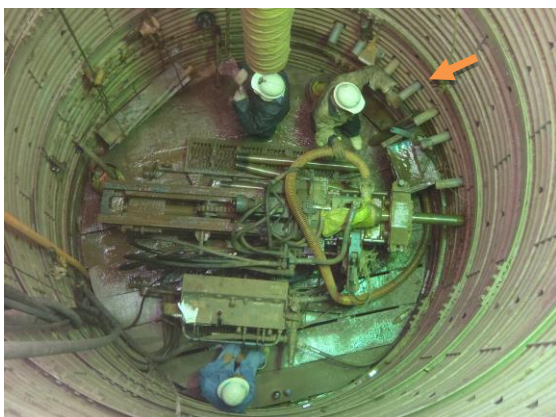
Fig. 7 Drilling of intake pipes. (Taken by Froilán Castro, 2013)
