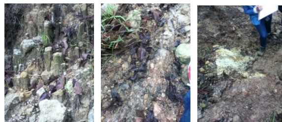
Fig. 8 Material detached due to the landslide
