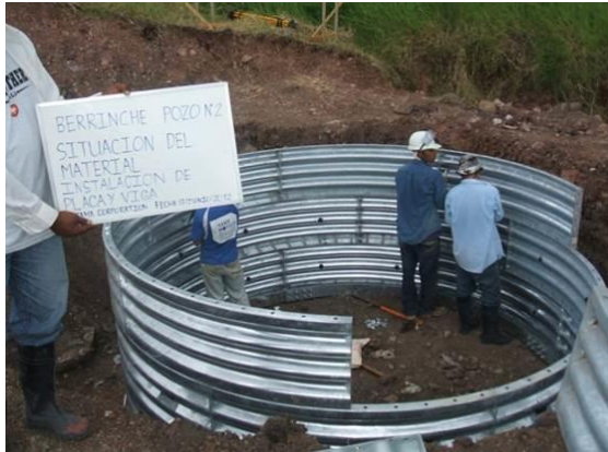
Fig. 6 Liner plate installation. (Taken by Froilán Castro, 2013)
