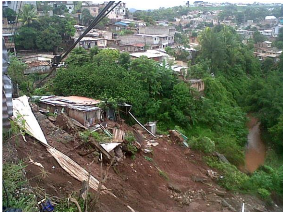
Fig. 2 The Izaguirre neighborhood suffered a landslide episode in 2014. Several houses were damaged and many inhabitants were affected. (This image is courtesy of El Heraldo newspaper.)
