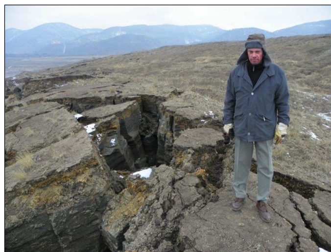
Figure 6 Head scarp in stiff-fissured clays under 190 m asl. (foto: Burda, January 2013).
