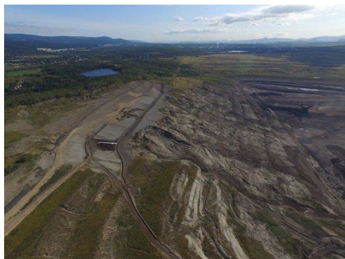
Figure 4 An aerial view on the Albrechtice landslide. In the left site is remarkable up to 10 m high head scarp. In the middle stabilization ground works and original landslide relief (head scarps, earthflows, tension cracks, etc.) in the lower part of the slope (foto: Burda, June 2015).
