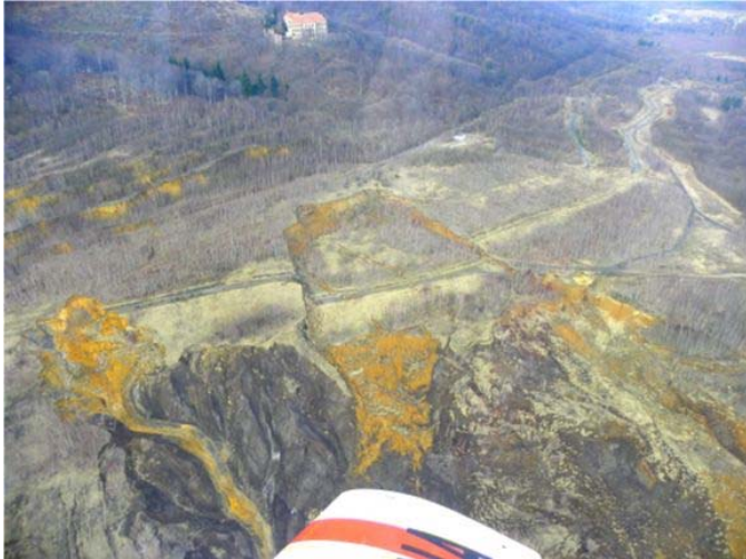
Figure 7 An aerial overview of the landslide complex situated at the edge of the open-pit mine (foto: Burda, January 2011).
