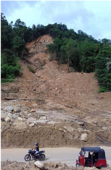
May 2017 Athwelthota landslide in Kalutara District Sri Lanka, which killed 09 people. Landslide was initiated from residual soil origin.
