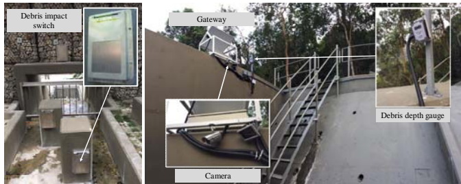
Figure 10 Trial field installation of Smart Barrier System
