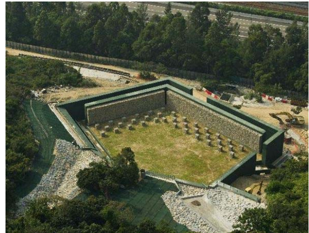
Figure 1 Rigid debris-resisting barrier constructed in Hong Kong
