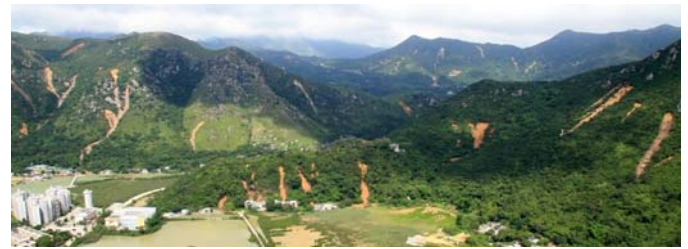
Figure 7 Multiple landslides occurred in Lantau, Hong Kong in 2008
