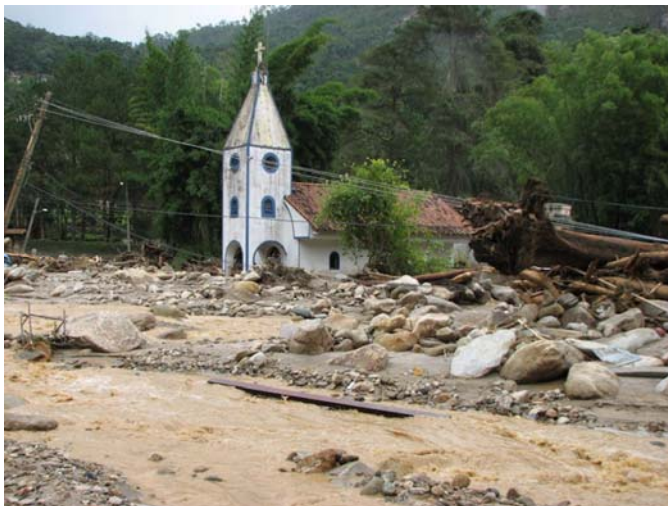
Figure 9 - Church in rural area of the city of Teresópolis affected by flow type mass movement in the State of Rio de Janeiro.
