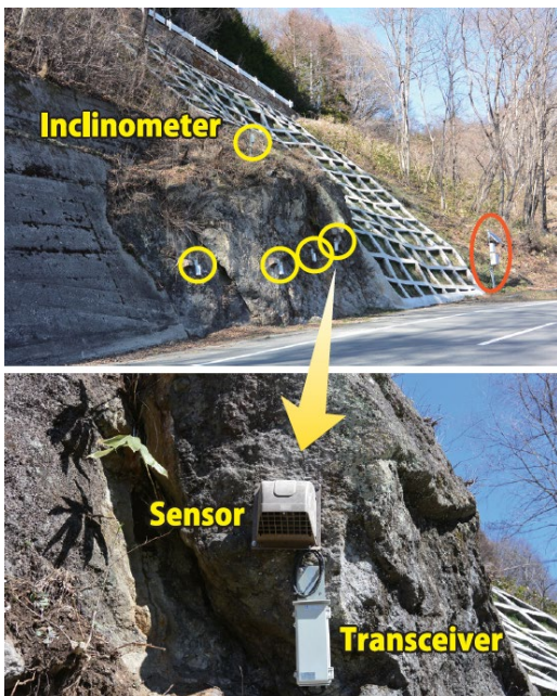
Fig1. Bedrock slope monitoring (maintenance control)
