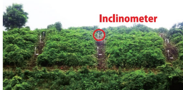
Fig3. Cut slope monitoring
